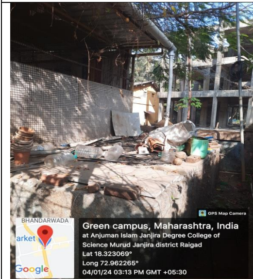
Rain water management
